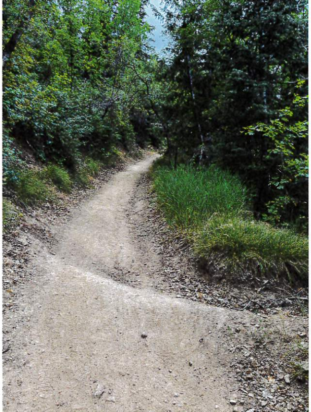
Water bars across the Switchbacks are necessary to push water off the trail.
